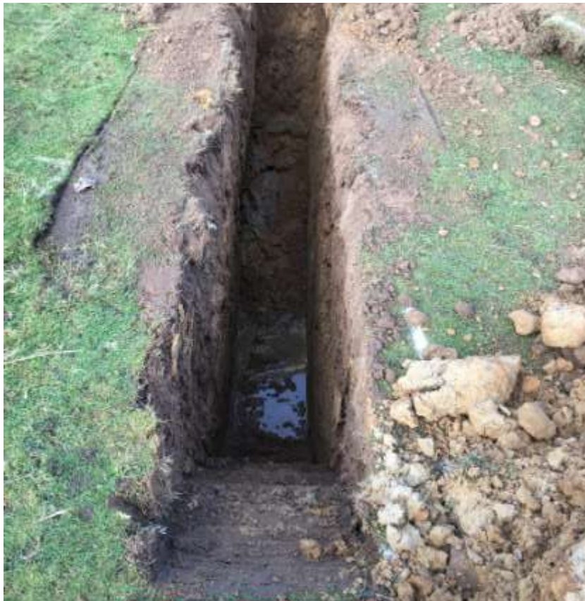
Plate 4: View of interim trench (looking north west)
